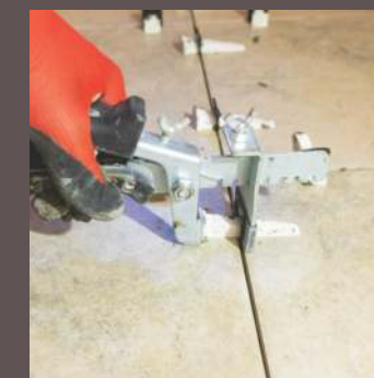
Levelling Wedges
