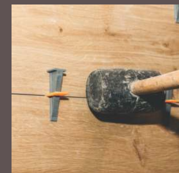
Remove Wedges Ones It Dry
