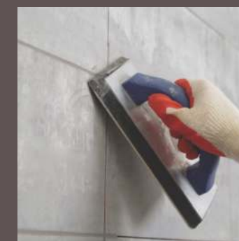
Joint Grouting
