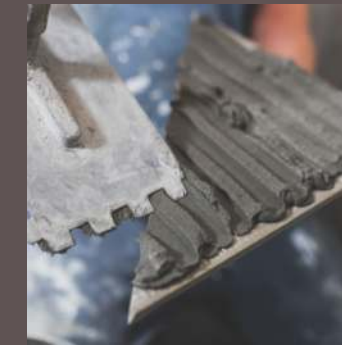
Cement Laying On Tile
